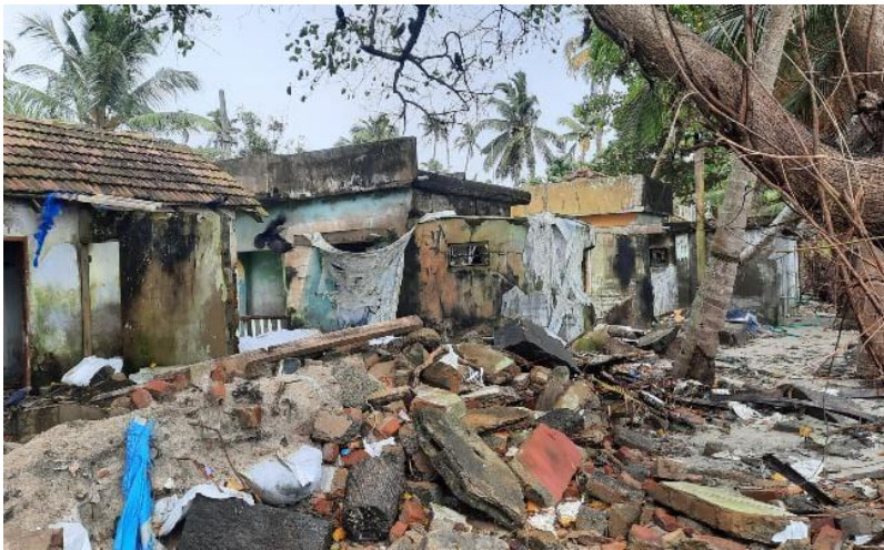
Pic 11: House destroyed due to Coastal flooding in Nayarambalam, Vypin
