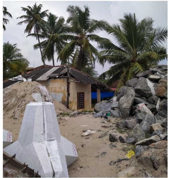
Pic 6: House being destroyed by the stone from seawall coming along the waves. Tetrapod came seen nearby
