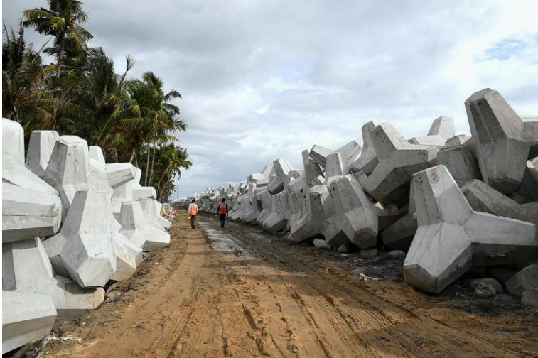
Pic 9: Construction of Seawall using Tetra pods
