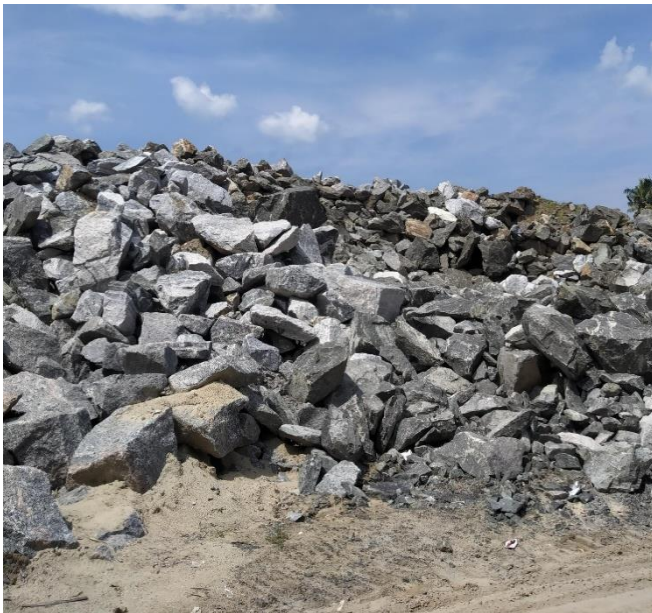
Pic 7: Construction of seawall in Chellanam
