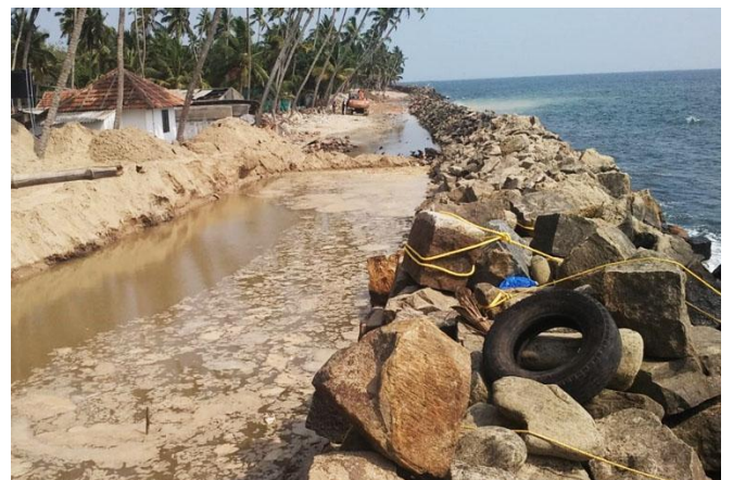
Pic 8: Clearing the water and constructing seawall using large stones
