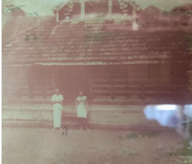
Pic 7 Naadagashaala before its demolition
